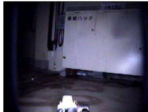
Check of the leakage from the equipment hatch
