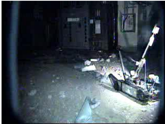
Picture from 1 st Floor Reactor Unit 1
